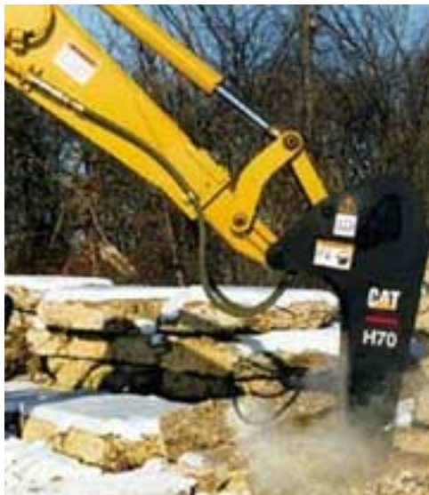
Skid Steer with Hammer
